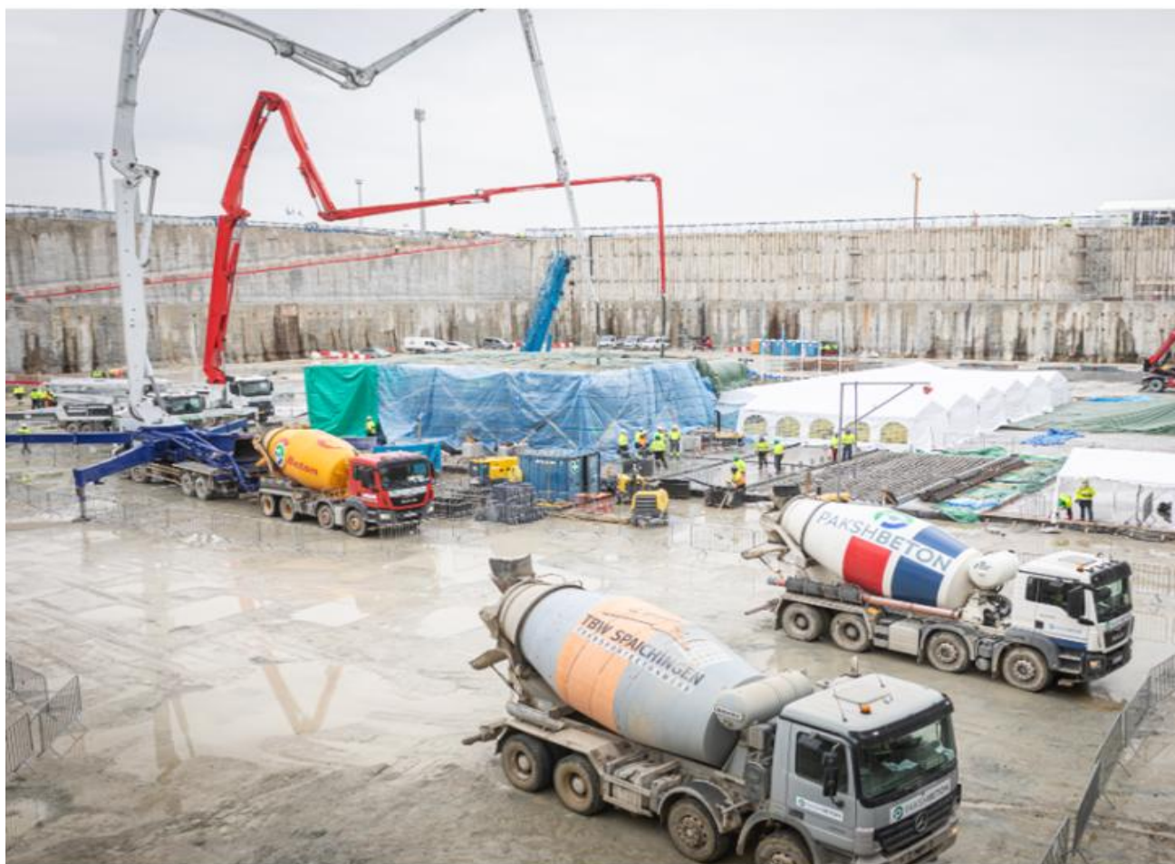
First concrete pouring at Bay 1.1 of the foundation slab for the Control building of Unit 5
